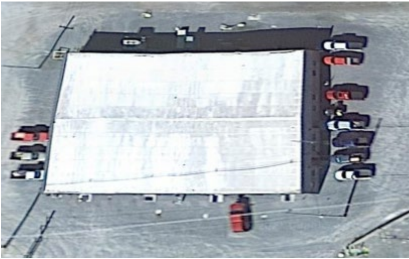
Acid / Prill Production Control room
