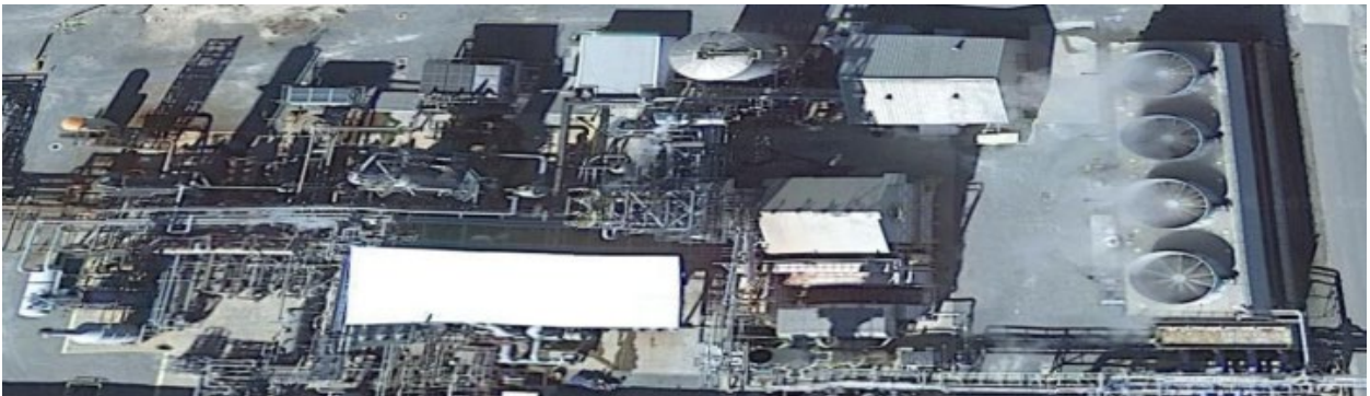
EDCC Ammonia Plant
